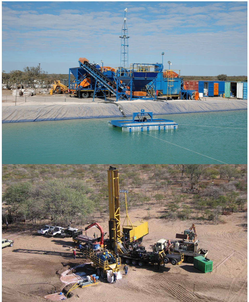
TOP: The BK16 kimberlite Dense Media Separation processing plant.
