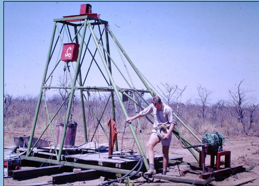
1968: 120ft deep evaluation pit samples to DMS plant
