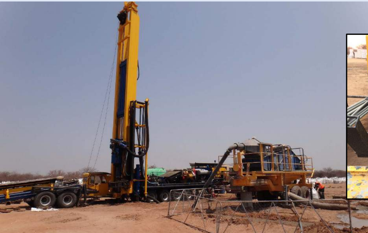
Elephant rig with on site 1 mm screening plant
