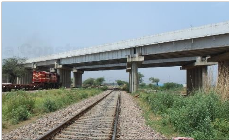
Figure 8-10: Road over Bridge
