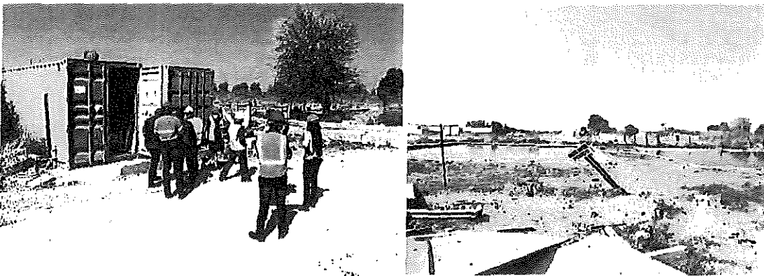
Figure 6 Wastewater Treatment Plant
