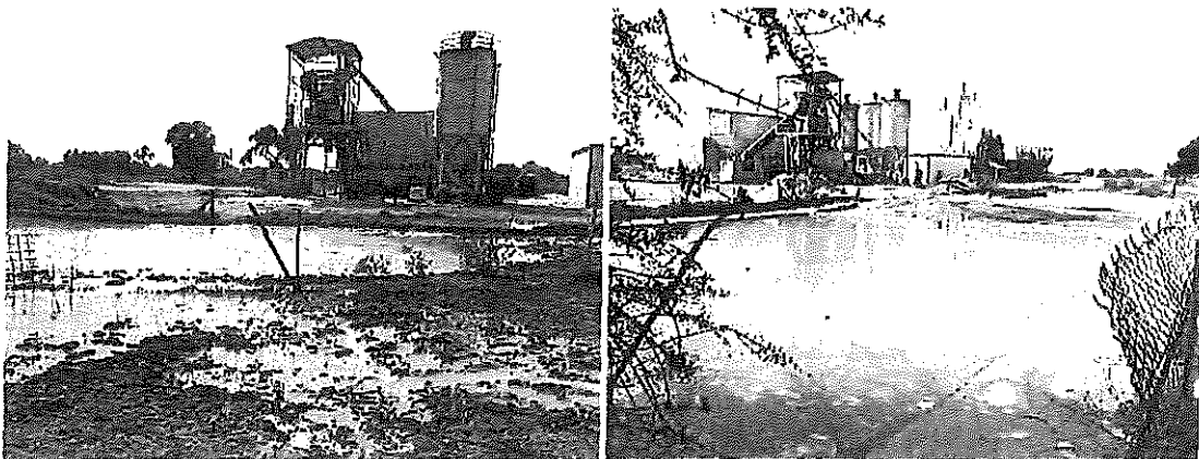
Figure 7. Liquid waste management at Cement-batching Plant
